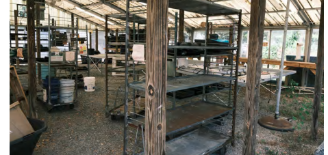
Interior of current greenhouse
